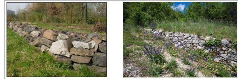
Figure 287: Muret de pierres sèches favorables aux reptiles
